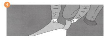
Using the trimmed edge of the first as a guide cut the edge, as above, and remove the surplus.
