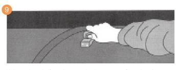
Using a sharp knife or Araseur trim the carpet to fit against the perimeter walls.
