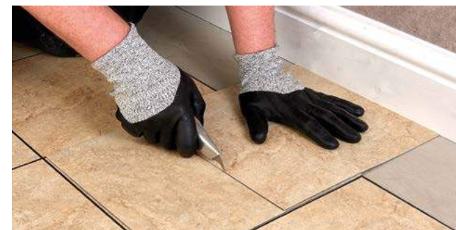
Figure 6 Measuring using an overlapping tile
