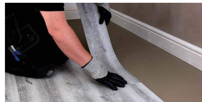
Figure 1 Setting planks out
