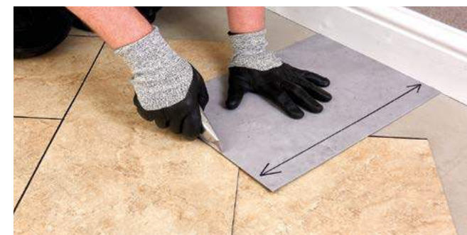
Figure 9 Cutting the perimeter tiles (diagonal cut)
